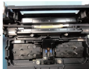
3. protection sleeve shrinking
